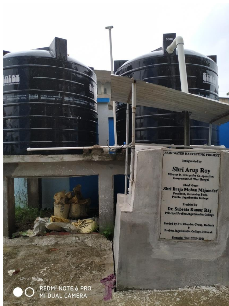
The Rainwater Harvesting Plant in Prabhu Jagatbandhu College
